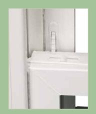
Vent stop, when deployed, will limit sash travel to allow for ventilation while still providing a degree of safety.
